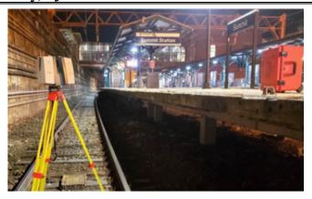
GEOD utilized a combination of conventional survey and 3d laser scanning to provide topographic basemapping to support the engineering for wall rehabilitation and drainage improvements at the Summit Station in Summit, NJ.
