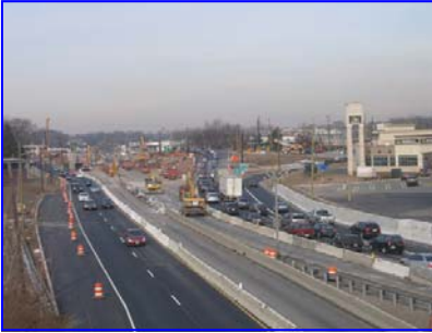
Essex Street Bridge over Route 17, Lodi, Maywood & Rochelle Park, NJ
