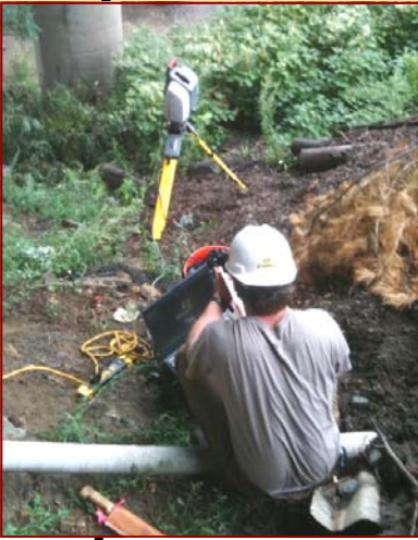
Laser Scanning the Tappan Zee Bridge
