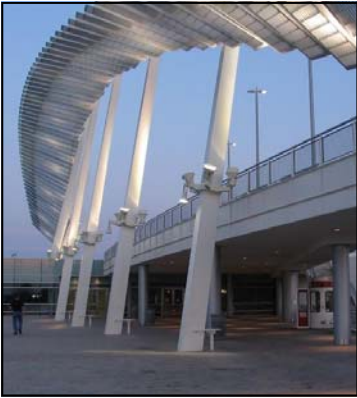
Ramp rehabilitation project at St. George Ferry Terminal
