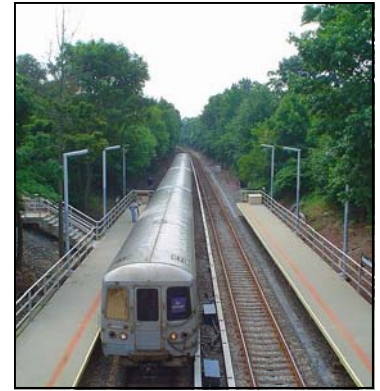
Staten Island Rapid Transit—Annadale
